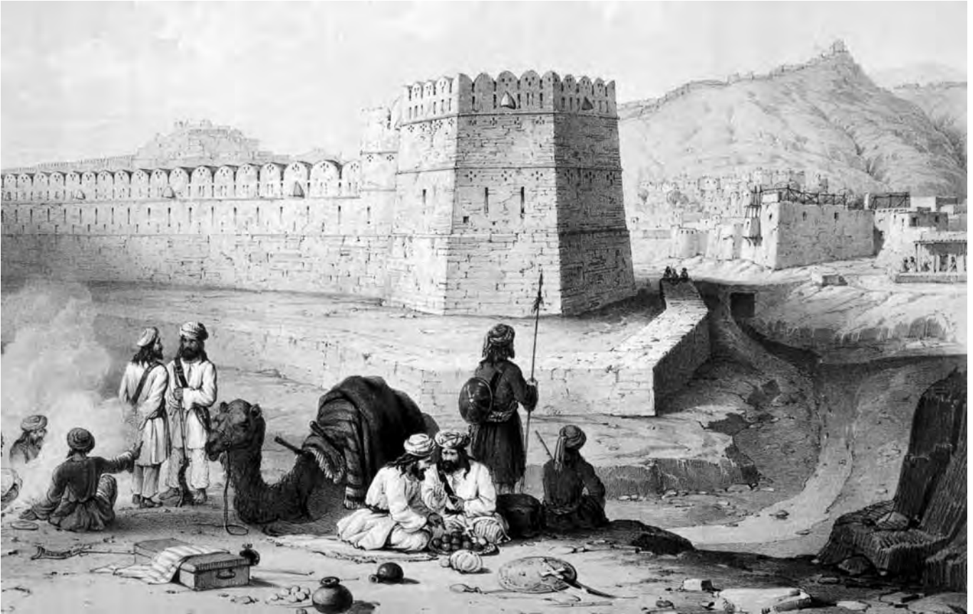
Figure 12. The north-west corner tower of the Bala Hissar. This was possibly drawn by Lieutenant Sturt between 1839 and 1841. 45 [Afghanistan Institute, Switzerland.]
