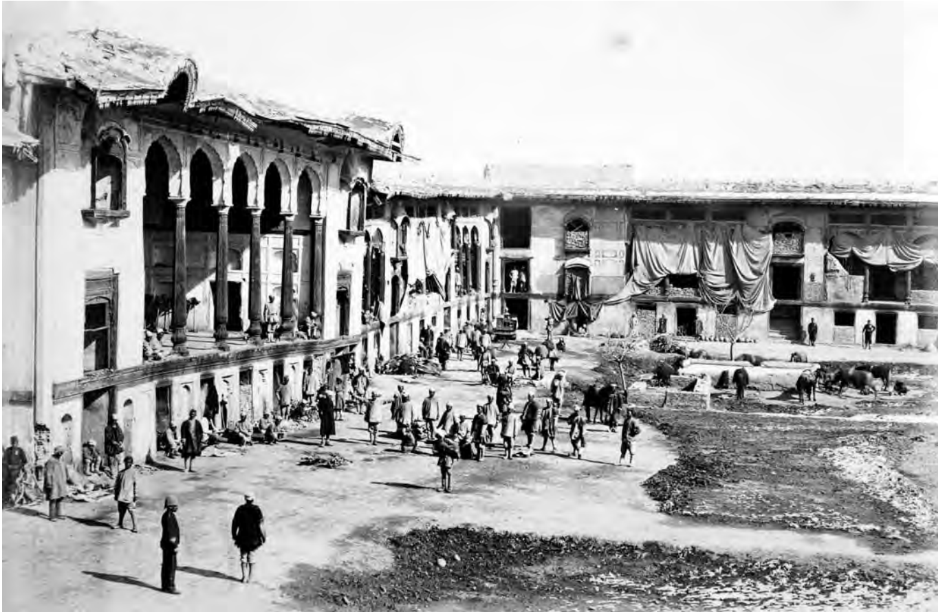
Figure 20. The courtyard of the former royal palace in the lower Bala Hissar. This photograph was taken in 1879 or 1880 when the palace area was occupied by a Gurkha regiment. The canvas shrouds were either hung to provide shade or protection from winter cold. The buildings have a basement storey (with kitchens, store rooms, servants rooms, etc) above which was the main level, with verandas interspersed with living quarters. These could also be on a floor above. [ Bengal Sappers & Miners; Institution of RE ]
