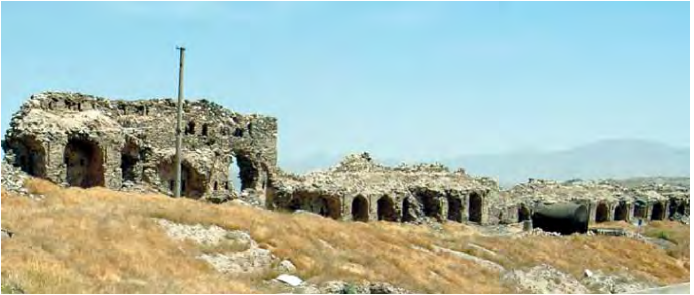
Figure 10. The interior of the walls on the north side of the upper Bala Hissar, probably of the Mughal period. [Author.]
