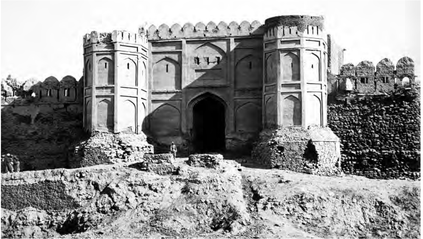
Figure 15. The Darwaza Naqqara Khana , also called “City Gate”. The top of the right-hand tower appears to have been re-fortified, possibly British work from 1880. [ Bengal Sappers & Miners; Institution of RE ]
