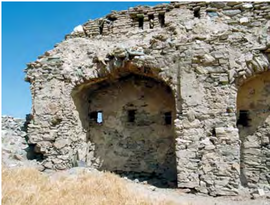
Figure 11. One of the probable Mughal-period casemates on the north side of the upper fort. The parapet above has angled firing loops. [Author.]
