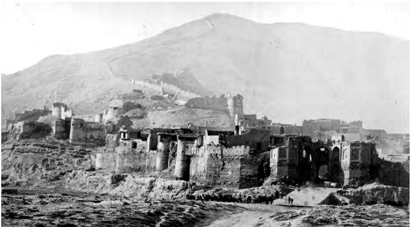
Figure 31. The south-east corner of the lower Bala Hissar in 1879, with the main gate on the right. The walls had become fairly degraded by this time and parts could not be used as a firing platform as buildings had been constructed on them. [Bengal Sappers & Miners; Institution of RE]
