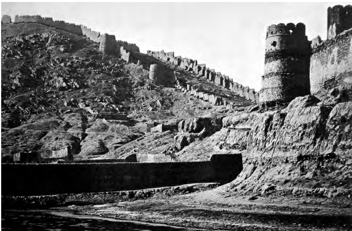
Figure 49. The partly-ruined walls rising up the hill to the west of the Bala Hissar to the Bala Burj. The wall at the bottom left of the photograph had no defensive purpose; it surrounded a vegetable garden. [Bengal Sappers & Miners; Institution of RE ]
